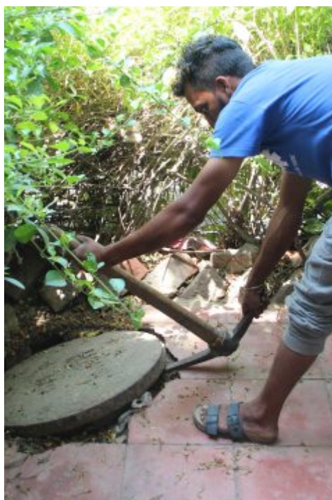
A sanitation worker is removing the lid from a manhole to work in it.
